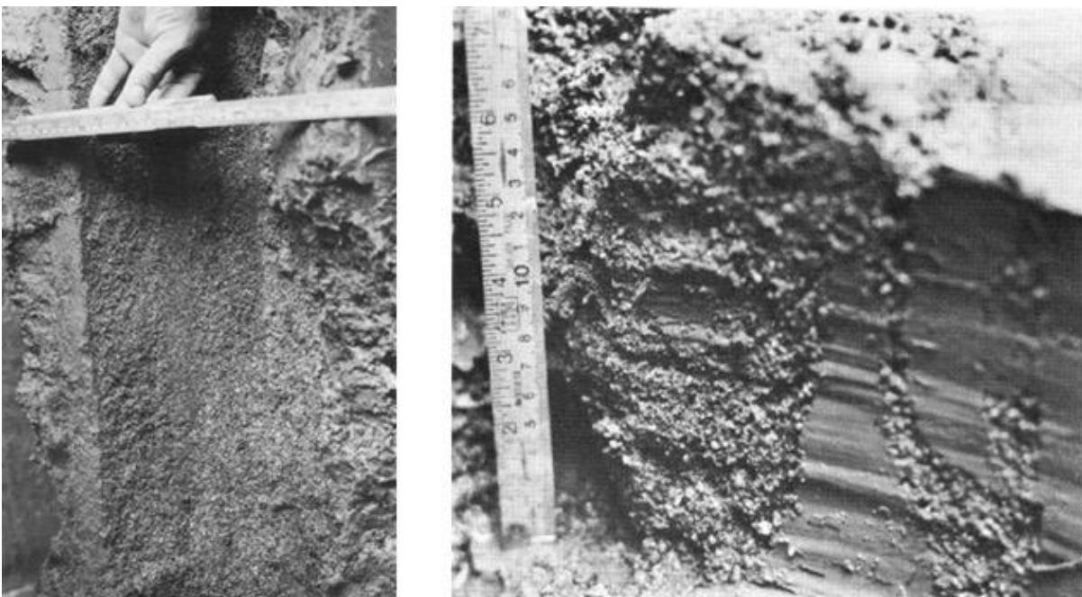
Figure 6. Sand-filled cracks adjacent to sand drains driven into soft clay, Holtz and Holm (1972).
