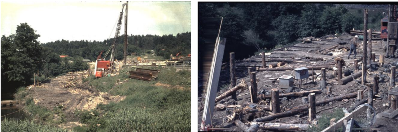
Figure 4. In-situ measurements during pile driving in clay at Nol, Sweden.
